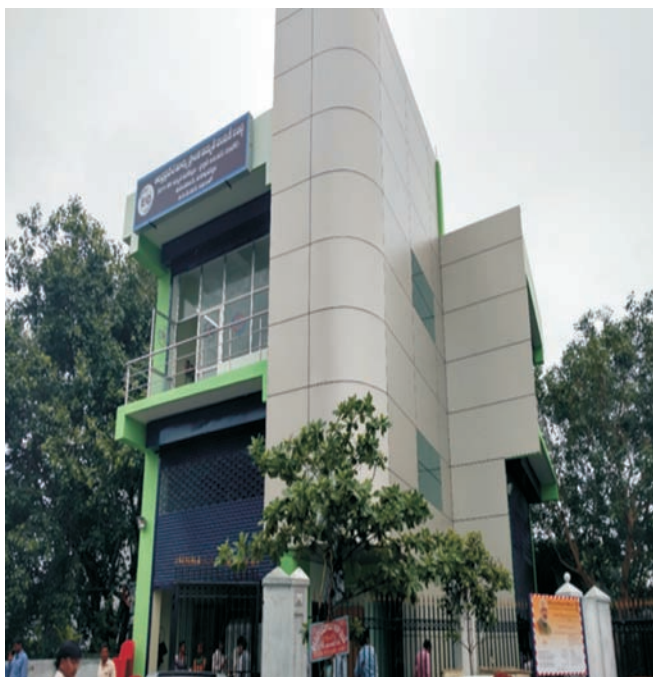
(Indoor Power Substation commissioned under IPDS in Andhra Pradesh)
