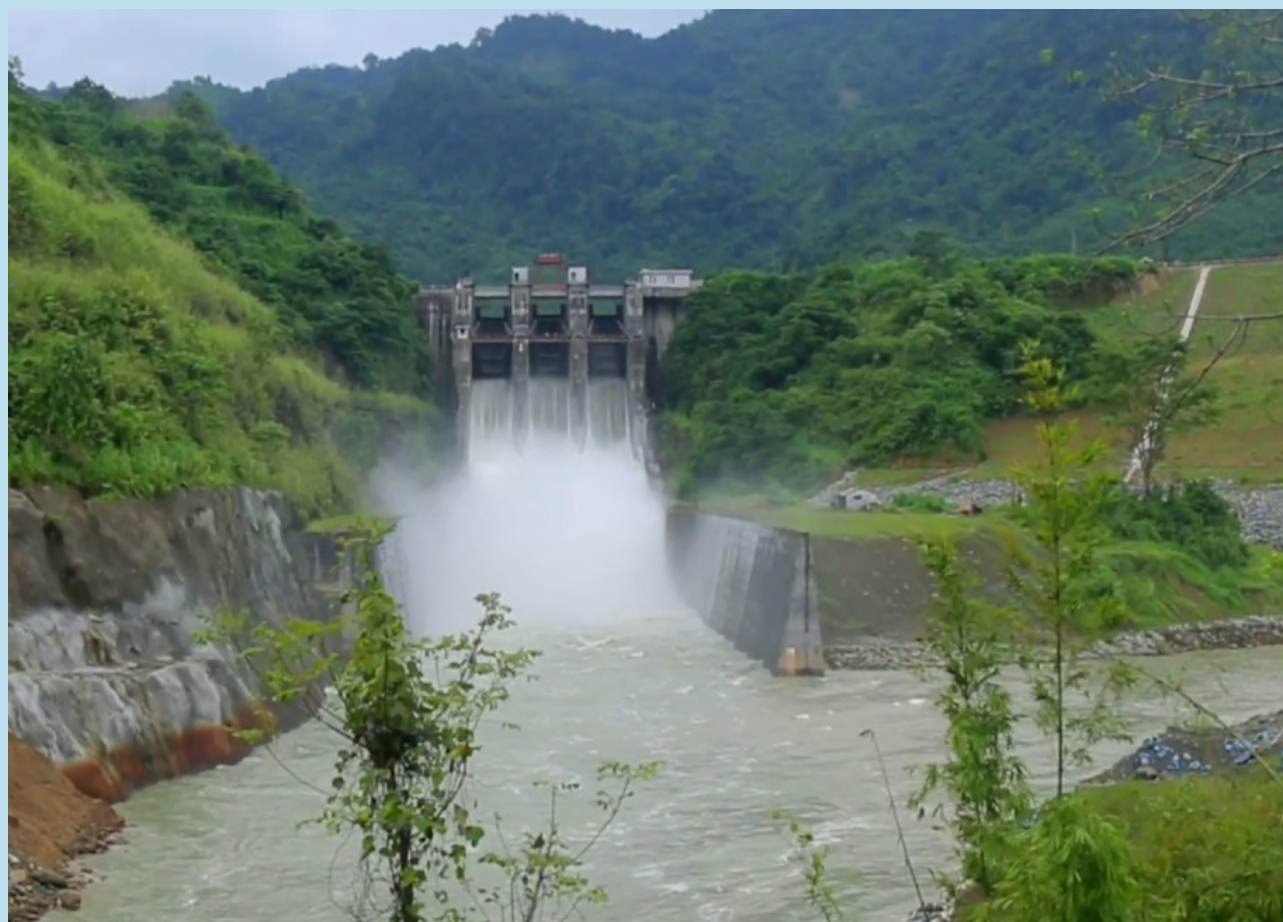
Tuirial Hydro Power Project, Mizoram
